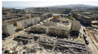
Photo 1 Effect of the earthquake in Boumerdes (Algérie 2003)
